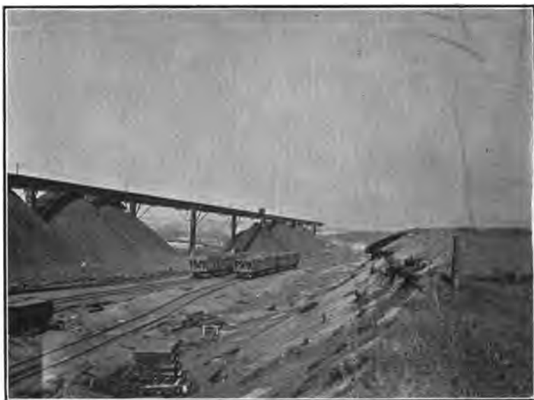
FIGURE 16 NEGAUNEE MINE TRESTLE
